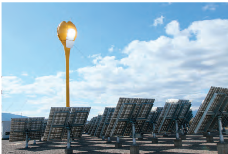
Aora Solar's solar tower in Almeria, Spain. Source: AORA SOLAR.
